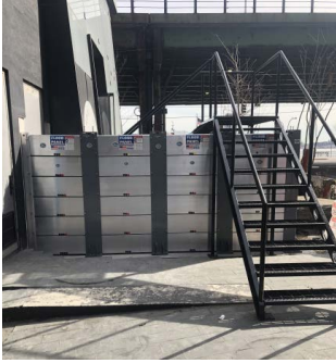
Emergency egress stairs
