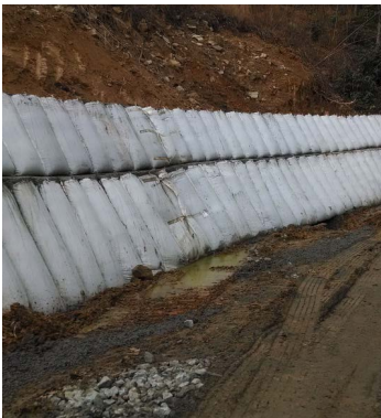
Roadside Levee Strengthening, KY
