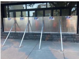
Vertical seam and support kickers
