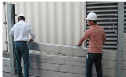
Deployment In Progress
