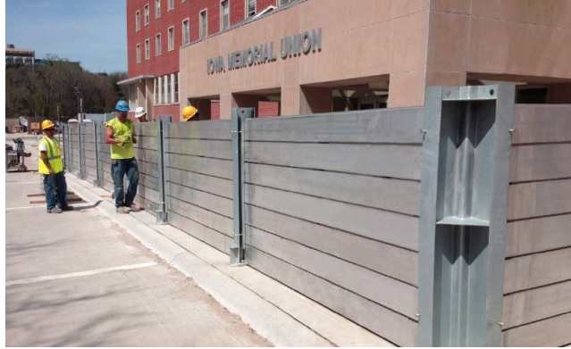
Corner Post Installation
