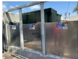
Custom support columns
