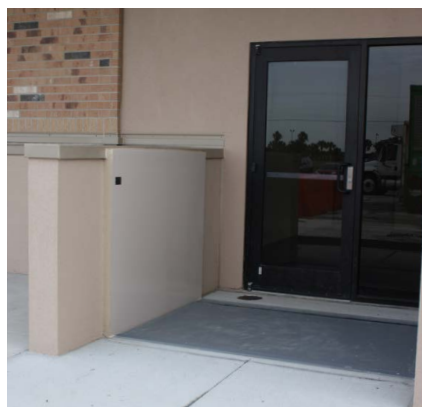
UTMB Primary Care Back Entrance, Galveston, TX
