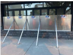
Vertical seam and support kickers
