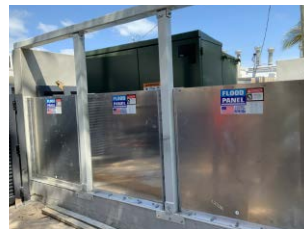
Custom support columns
