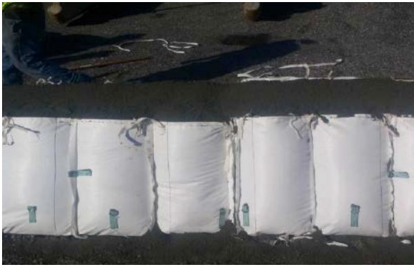
Connected 2' x 4' VersaShield Filled With Sand
