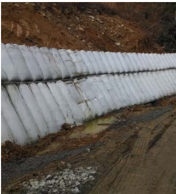
Roadside Levee Strengthening, KY
