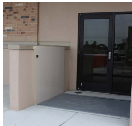
UTMB Primary Care Back Entrance, Galveston, TX
