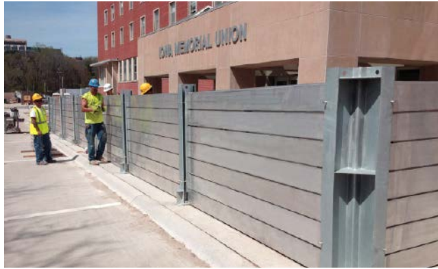
Corner Post Installation
