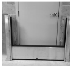
Stages of Set Up for Flood Logs. Color Coded For Easy Assembly
