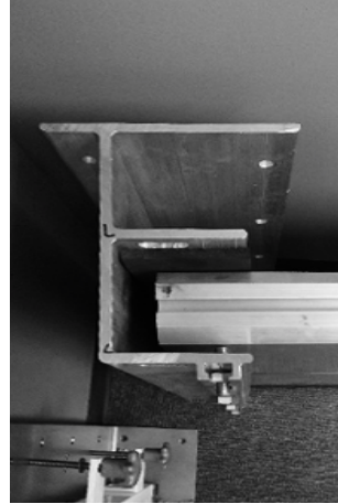
Offset Bracket Gives Wall Clearance
