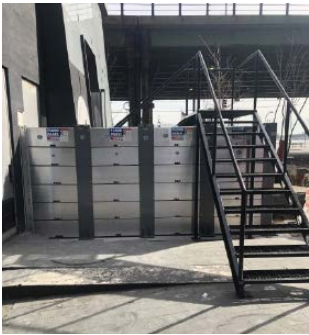
Emergency egress stairs
