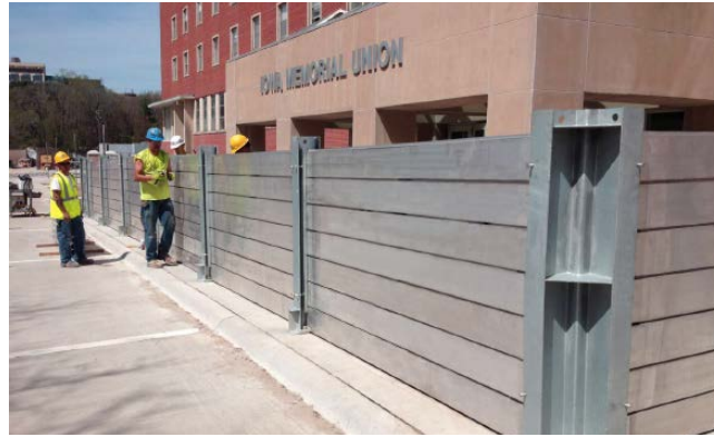
Corner Post Installation
