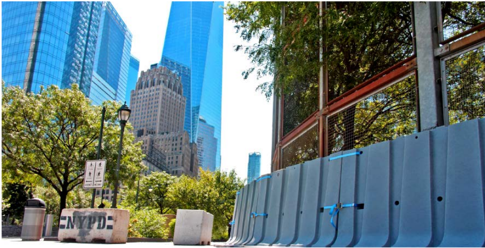
Muscle Wall Protecting Battery Park in New York City
