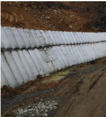
Roadside Levee Strengthening, KY
