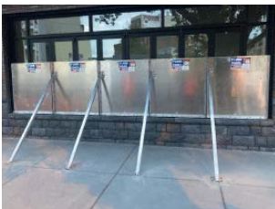
Vertical seam and support kickers
